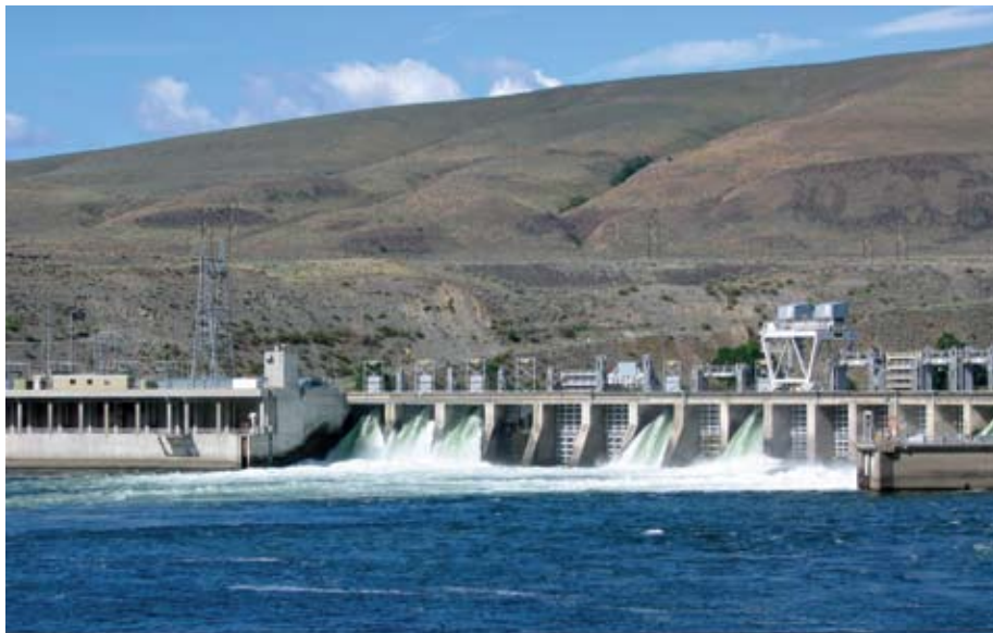
Hydroelectric dam in the Northwest
